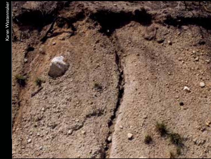
Erosion – Surface erosion.
