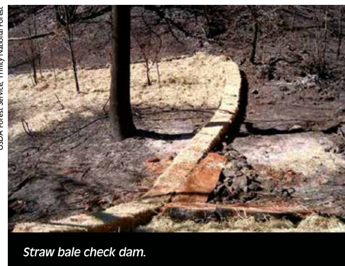
Failed straw bale check dam.
