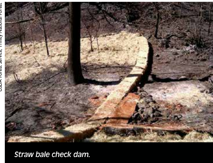
Failed straw bale check dam.
