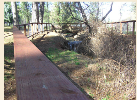
Fencing & erosion control
