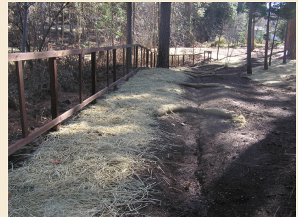
Erosion control and grading
