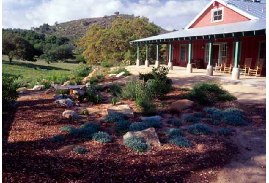
Figure 2: The 8 foot decomposed granite apron around this house has helped it withstand two major fire events in 2003 and 2007.
